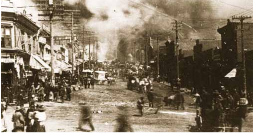
Towns built of wood often burned down. Two 1896 fires destroyed Cripple Creek. What damage can you see in this photo?
